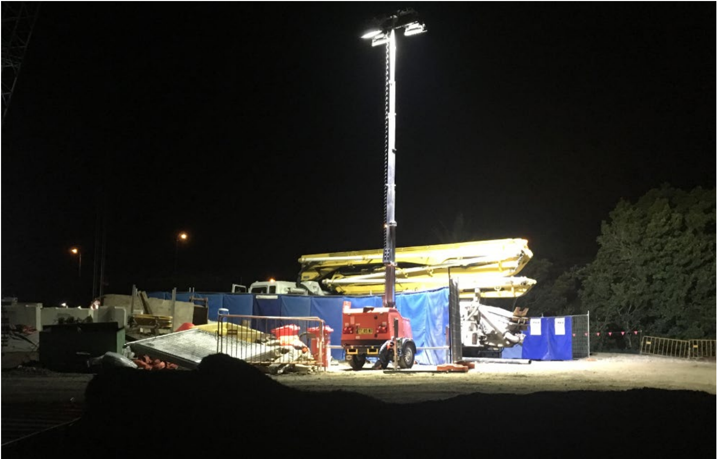
Above: Night works area with noise mats around the truck
